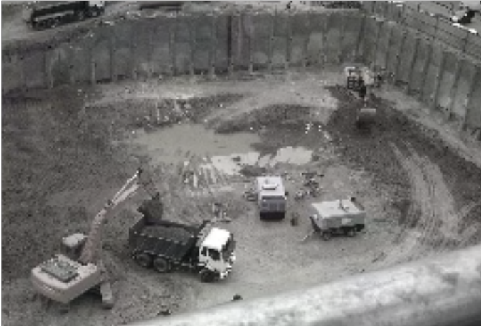
fig11 - City Property basement parking excavation
