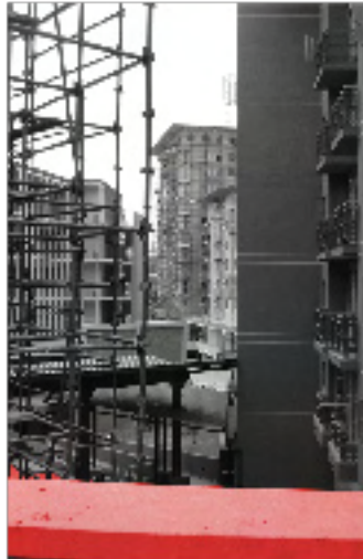
fig10 - City Property refurbishment
