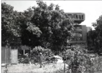
fig4 -Office building, northern boundary
