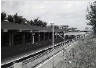
fig7 - Metro train track
