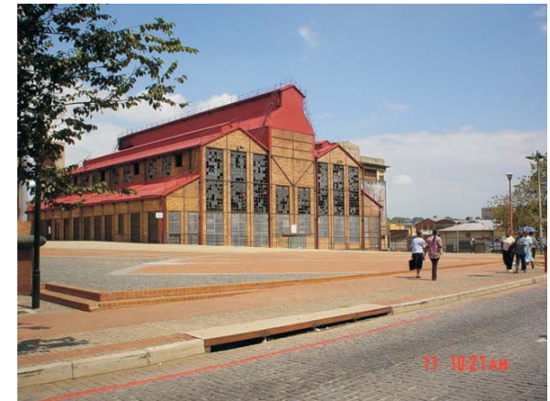
Fig 71. View to Turbine Hall from West Street.
