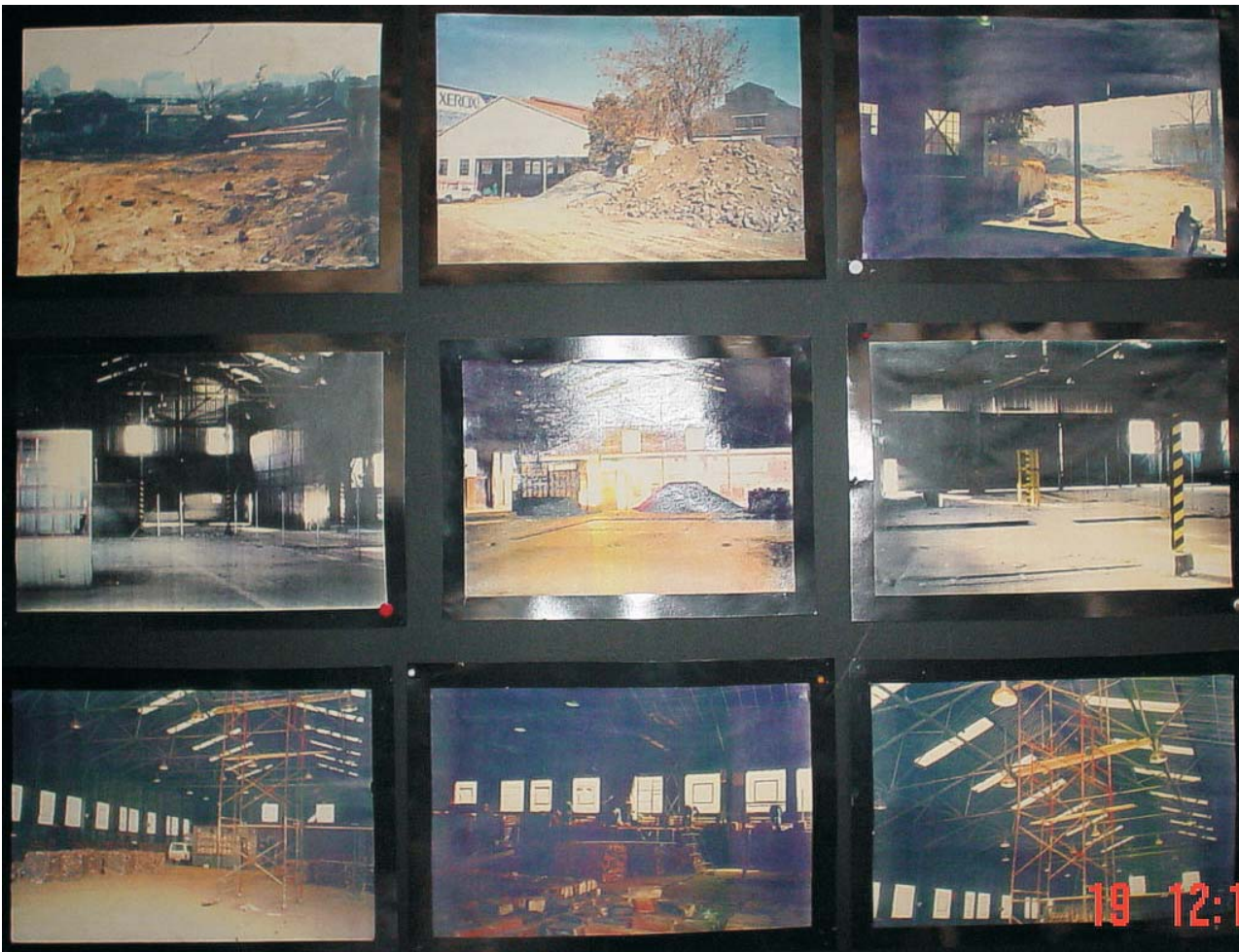
Fig 135. Renovation of the old warehouse.
