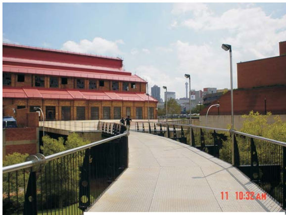
Fig 69. View to Turbine Hall from the pedestrian bridge.
