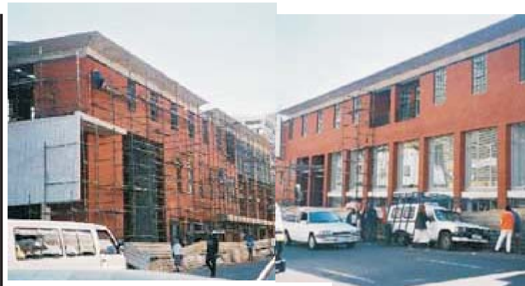
Fig83. The Metro Mall during construction.
