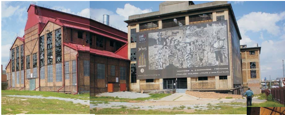
Fig 67. The Turbine Hall.
