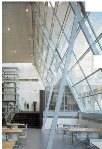
Fig 150. Light pours into the foyer through the huge sloping glass wall.
