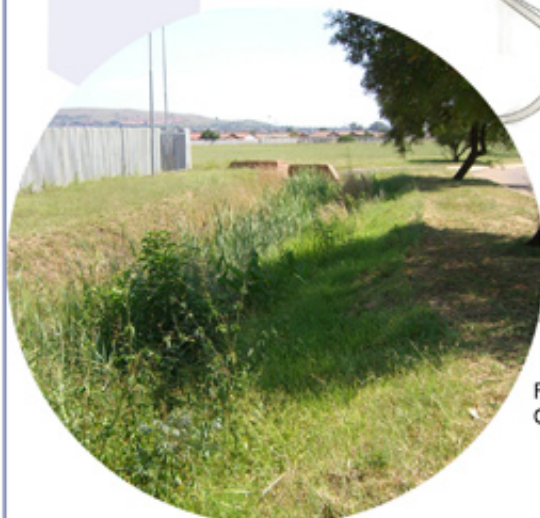
Figure 86: Storm water runs in a vegetation-lined permeable channel on the eastern side (Author, 2008)
