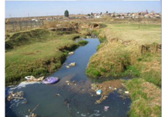
Figure 110: Water course - littered and eroded (Author, 2008)
