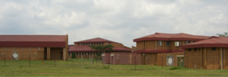
Figure 89: Northern elevation of the UP Mamelodi campus (Author, 2008)
