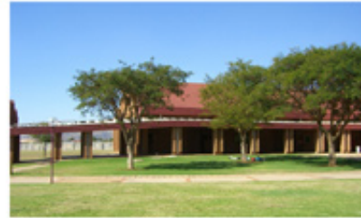
Lecture halls, presently in use - single storey
