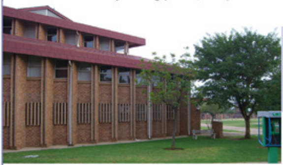
Figure 101: The library building is almost completely visually impermeable (Author, 2008)
