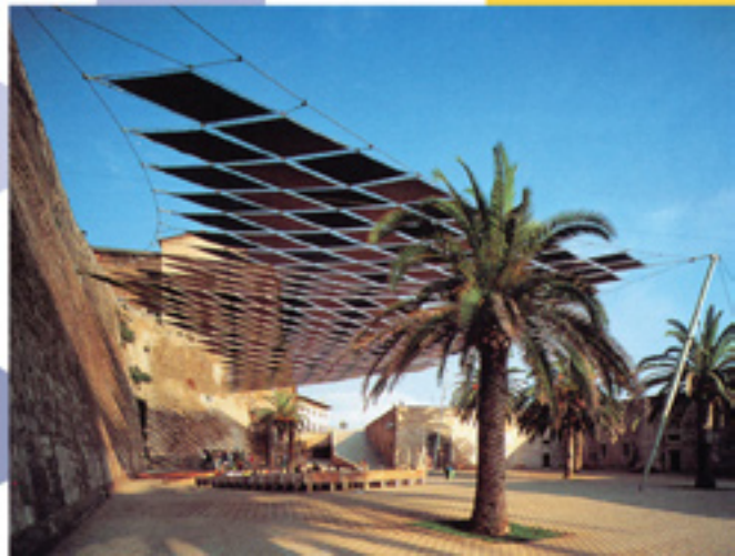
Figure 241: Shading structure (Unknown, [S.a.])
