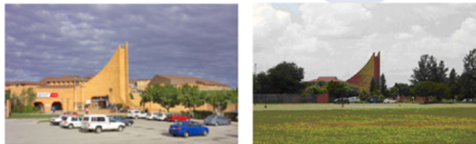
Figure 15 & 16: Landmark buildings on both the Port Elizabeth NMMU Vista campus and the UP Mamelodi campus are identical (Nelson Mandela Metropolitan University. www.nmmu.co.za , [S.a.]) (Author, 2008)
