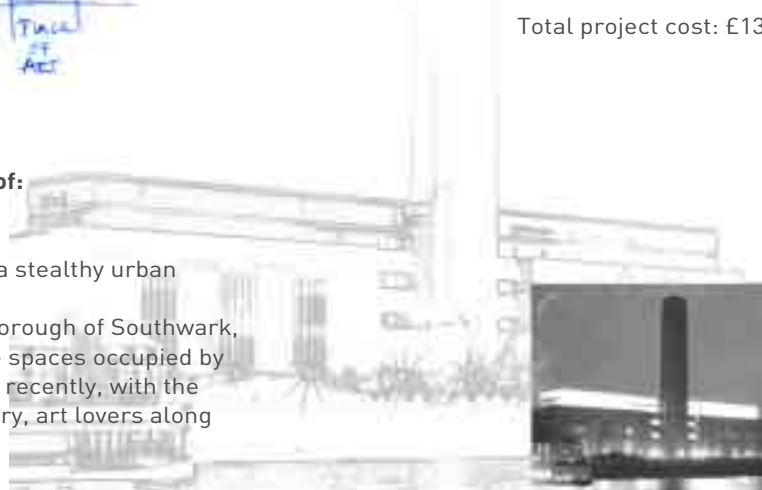
Figure C.1.3 Power station conversion
