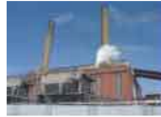
Figure B.5.5 East view of Power station B
