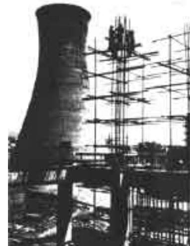
Figure B.5.11 The erection of cooling tower 2
