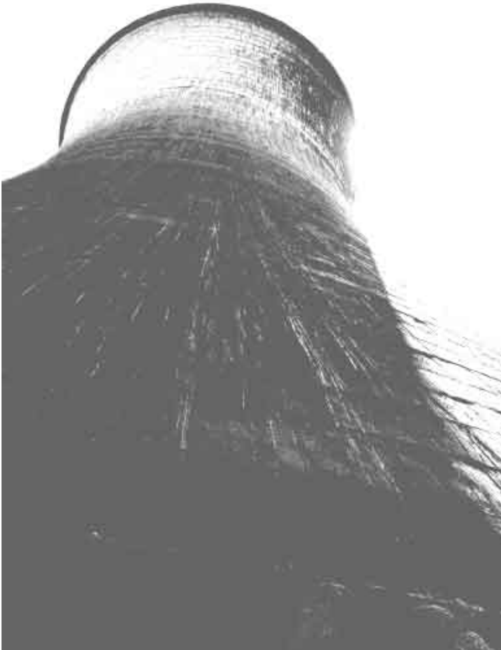
Figure A.1.2 Existing cooling tower
