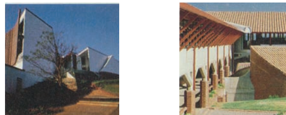
Figure 7.8: Photos showing the clay sunscreen and the terracotta roof tiles laid on asbestos
