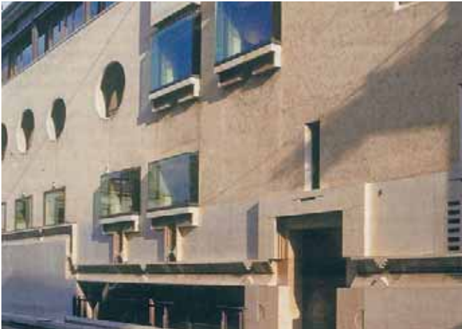
Figure 2.29: Facade facing Piazza Nogara. (Source: Schultz, 2010: 113)
