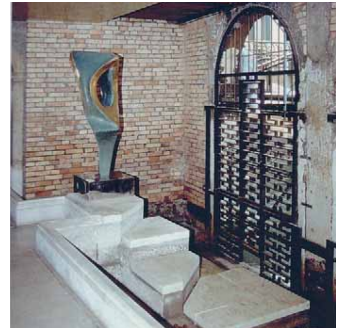
Figure 2.24: Water entrance, with concrete steps and stone treads. (Source: Schultz, 2010: 104)
