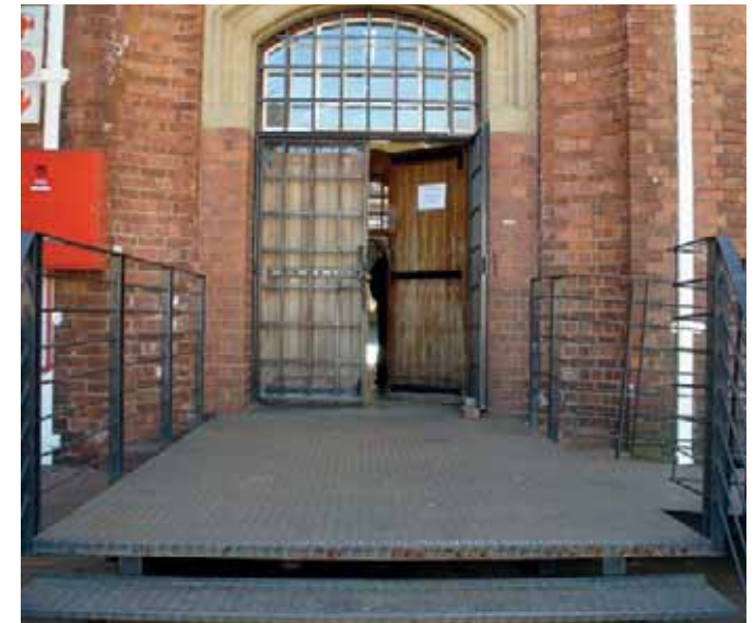
Figure 2.49: Existing main entrance with view axis into courtyard. (Source: Author)
