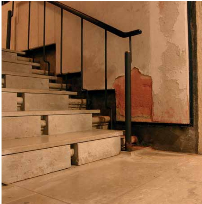
Figure 2.22: Stair cladding and stucco wall panels. (Source: Schultz, 2010: 108)
