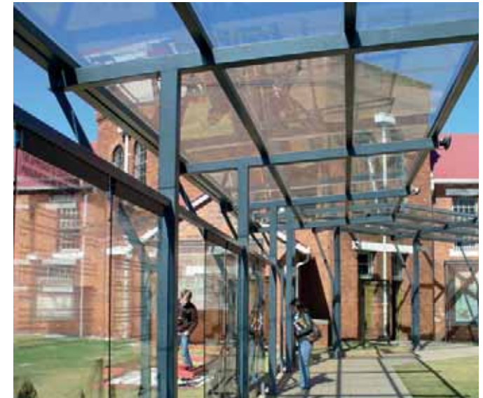
Figure 2.50: New covered walkway and axis in courtyard. (Source: Author)
