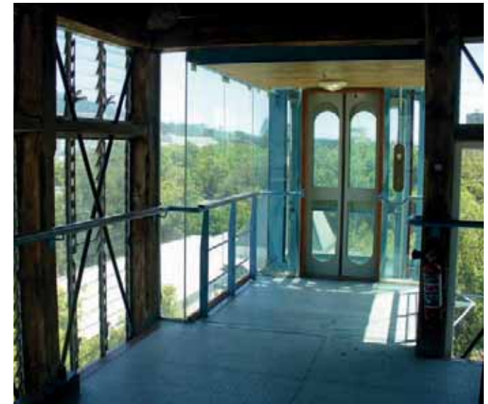
Figure 2.43: The new glass lift at the top of the tower. (Source: Author)
