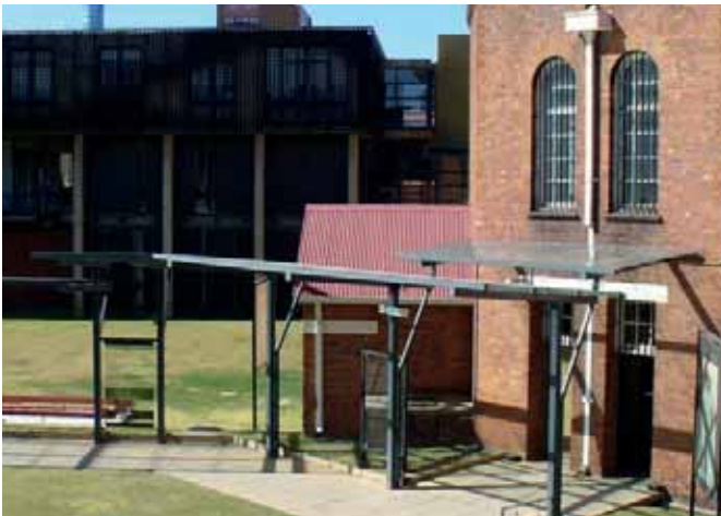
Figure 2.45: New addition on the left and the original building on the right with the new covered walkway. (Source: Author)
