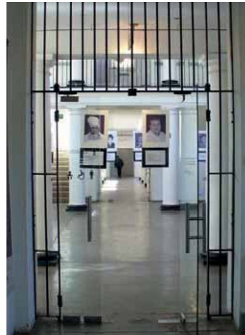
Figure 2.53: New frameless glass door layered in an existing steel door. (Source:Author)
