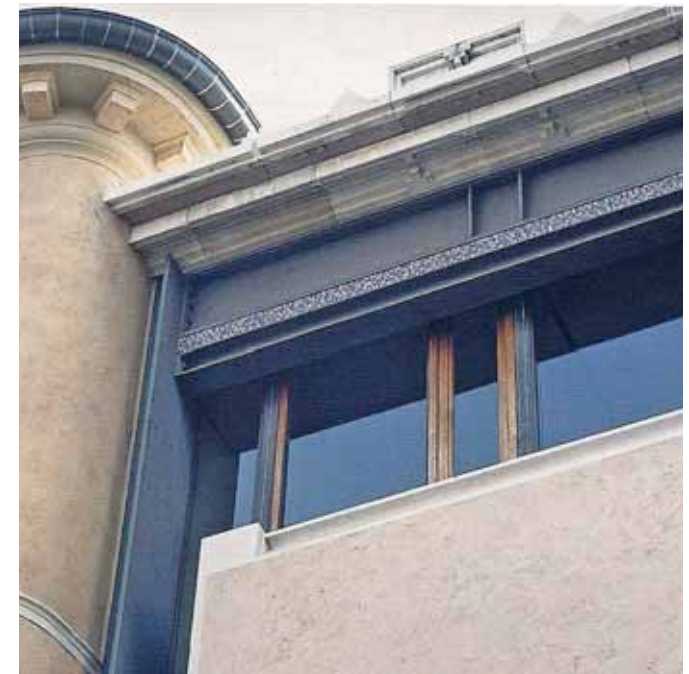
Figure 2.34: Facade joint to adjacent building with glazing detail. (Source: Schultz, 2010: 121)
