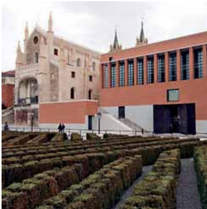
Figure 2.67: The new Moneo extension with the Jeronimos cloister incorporated. (Source: Arcspace)
