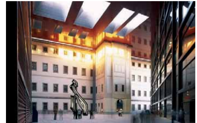
Figure 2.60: The original Sabatini building juxtaposed against Nouvel's new pavilions and aluminium roof. (Source: Architectural Record: 89)
