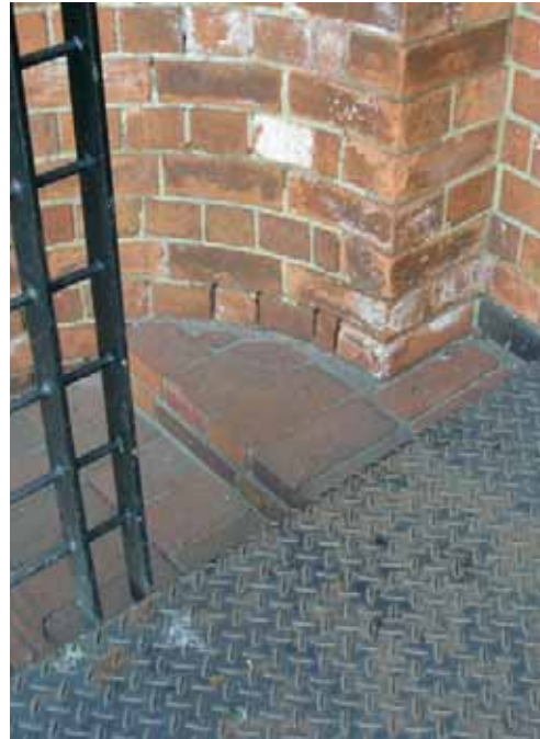
Figure 2.52: New steel ramps layered over existing steps. (Source:Author)
