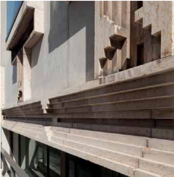
Figure 2.32: Stone cladding of the facade's Base Zone. (Source: Schultz, 2010: 121)
