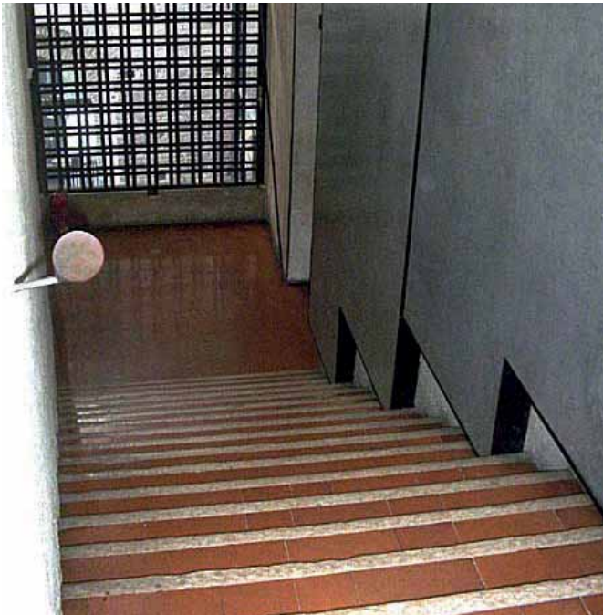
Figure 2.9: New stucco wall panels at staircase with the original wall finish still visible. (Source: Schultz, 2010: 94)
