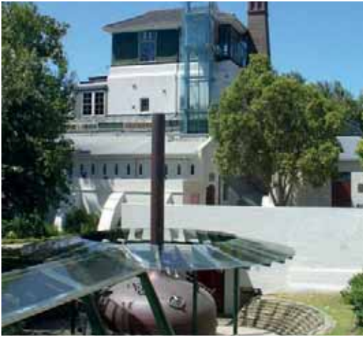
Figure 2.35:View of new link and glass lift. (Source:Author)
