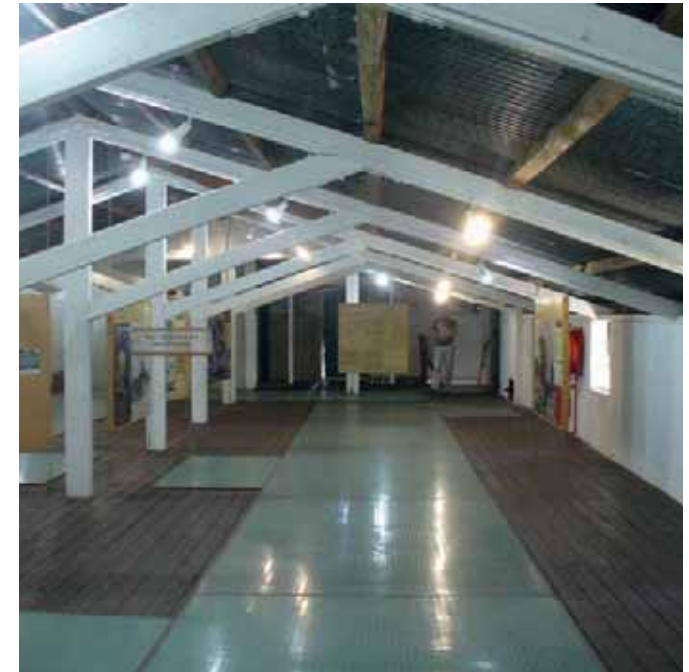
Figure 2.37: New floor finish layered over the old in exhibition space in Ohlsson's malt house (Source:Author)
