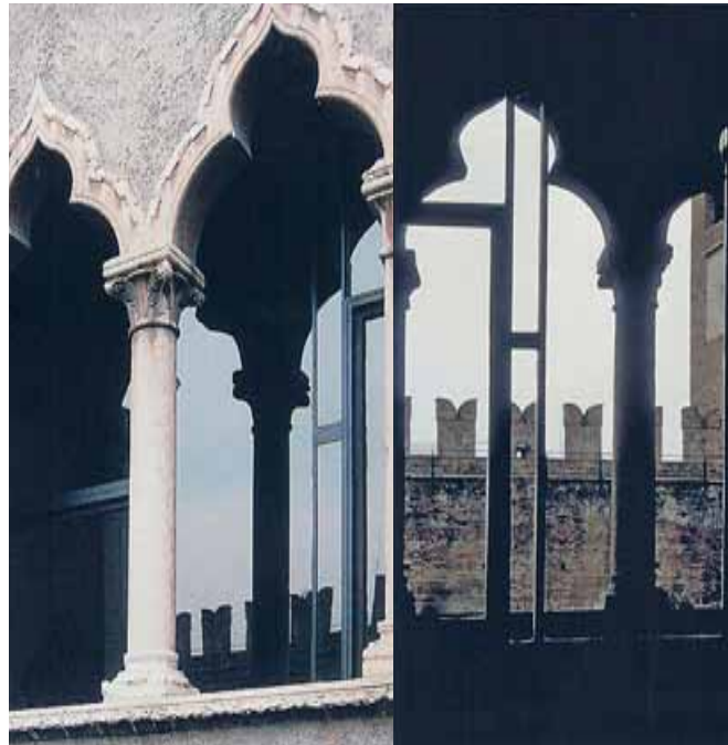
Figure 2.10: New windows set back from the original. (Source: Schultz, 2010: 92)
