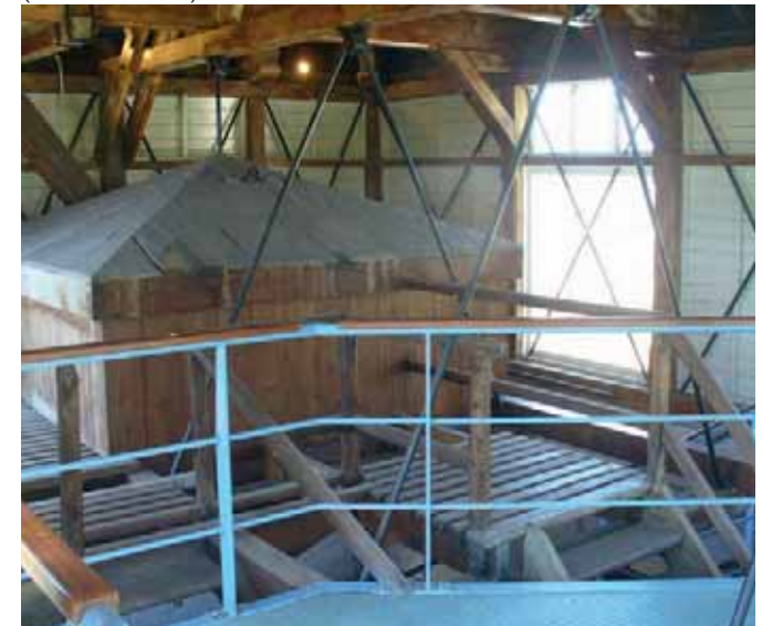
Figure 2.44: The new mild steel circulation route, painted blue, descending in between the existing. (Source: Author)
