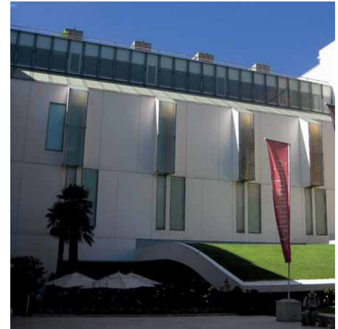
Figure 2.77: The new BOPBAA addition and café. (Source: BOPBAA)
