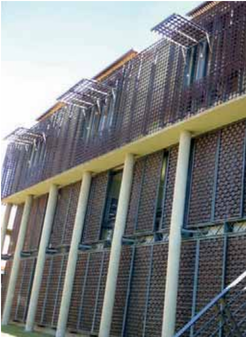
Figure 2.51: Facade with screen of new building. (Source:Author)
