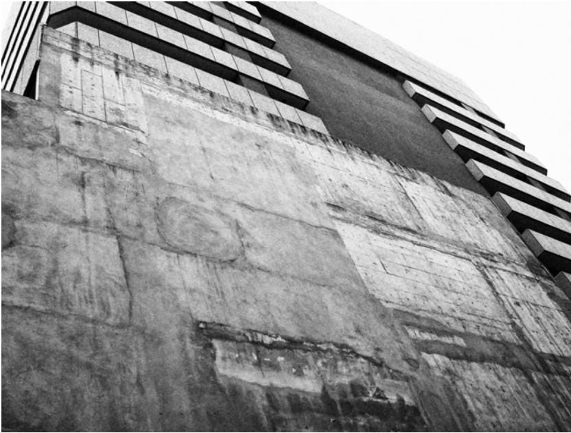
Fig. 3-31 Concrete scarring on Momentum facade facing site. (Photo by author).
