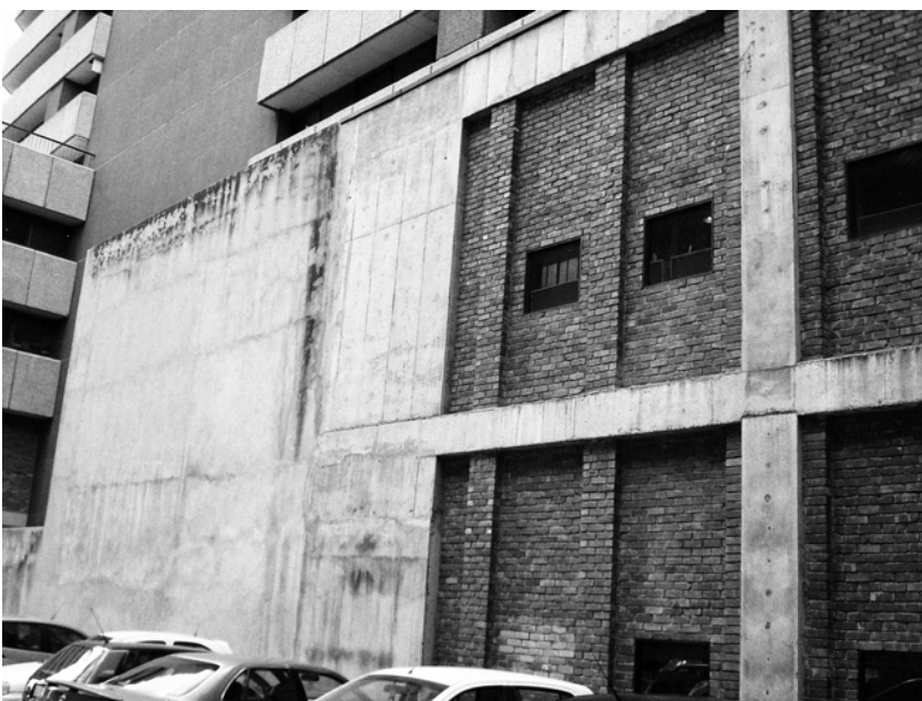
Fig. 3-30 Brick infill between concrete core structure of Momentum Centre, forming a barrier to pedestrian movement. (Photo by author).
