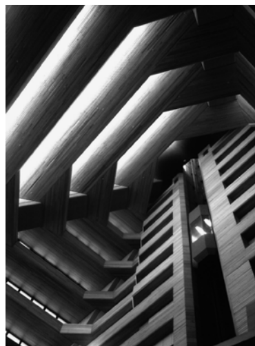
Fig. 3-60 (Bottom) Momentum Centre forum space lit by overhead skylight.
