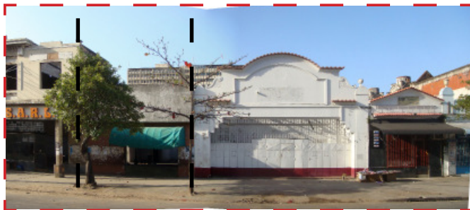
proposed demolition for new vehicular access
