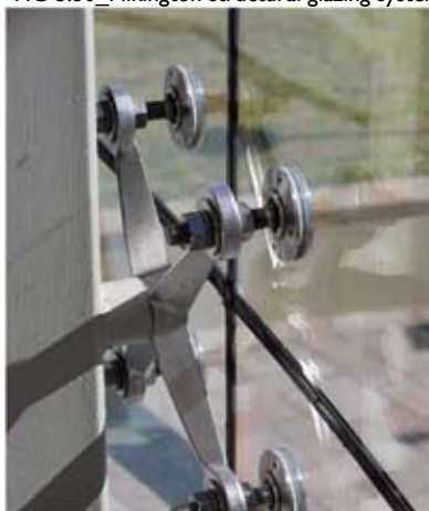
FIG 5.32_Glazing clamp detail
