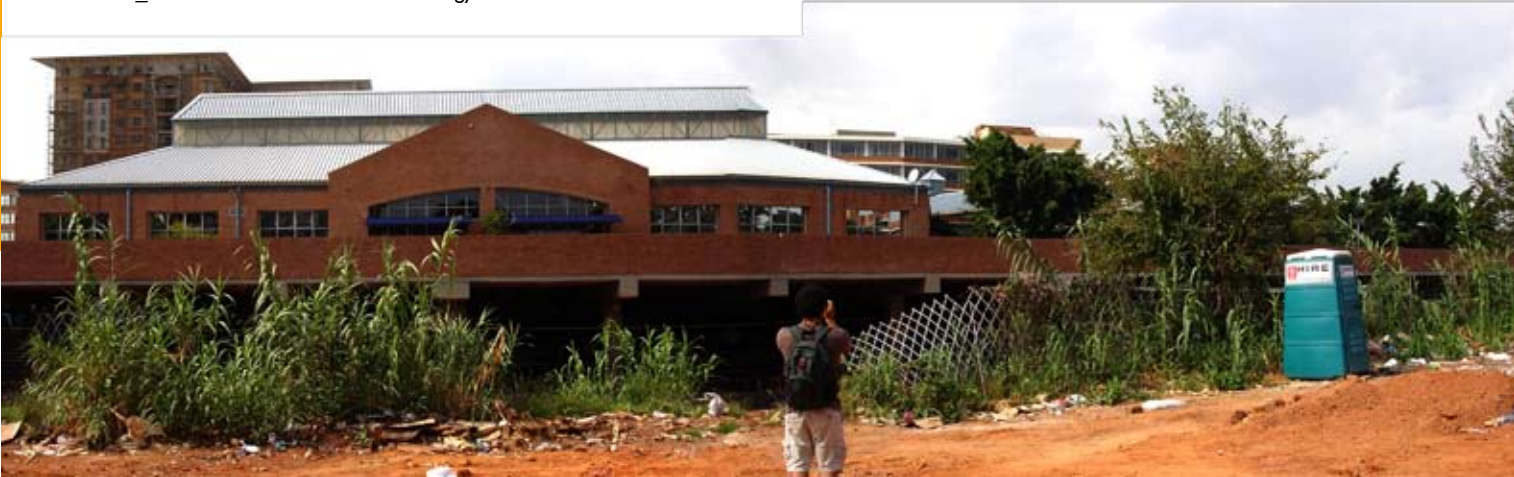
FIG 2.19_ Panoramic view from site towards gym
