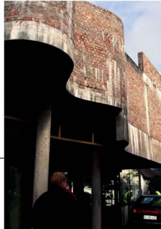
FIG 5.40_Weathered materiality of brickwork
