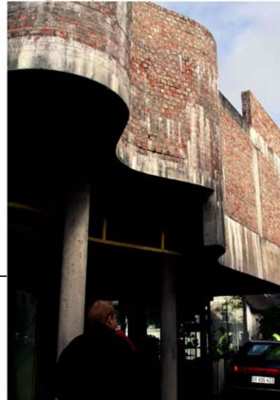
FIG 5.40_Weathered materiality of brickwork
