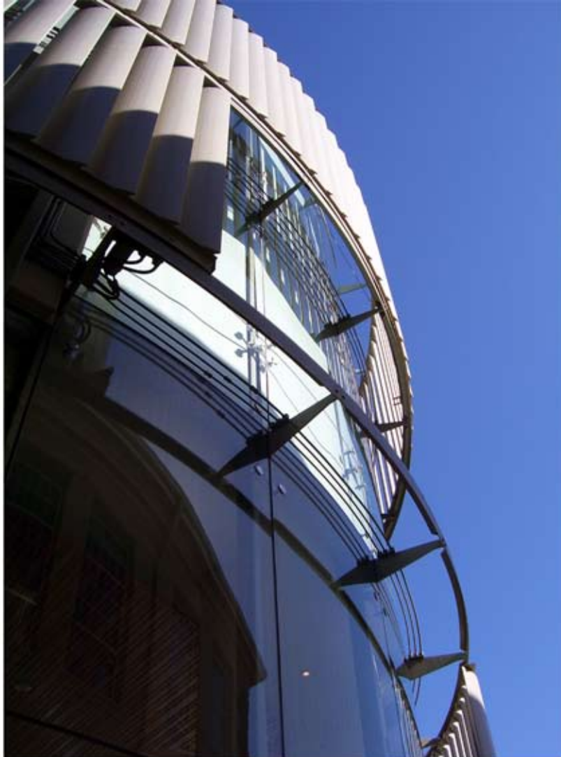
FIG 5.30_Pilkington structural glazing system with moveable shutters
