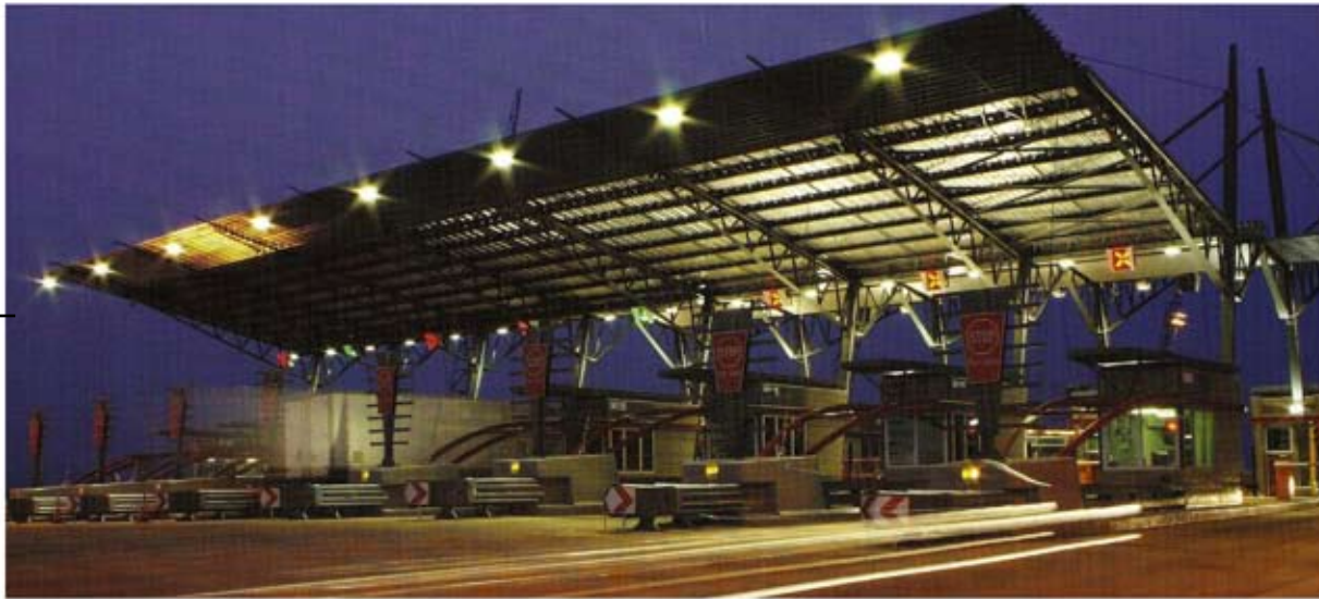
FIG 5.45_Industrial tectonic of exposed steel lattice trusses
