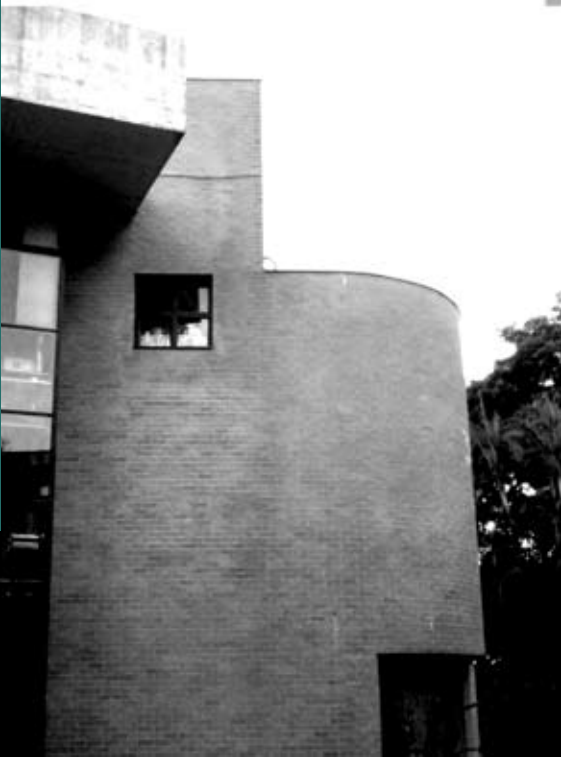
FIG 4.28_Opening placement enhances mass articulation
