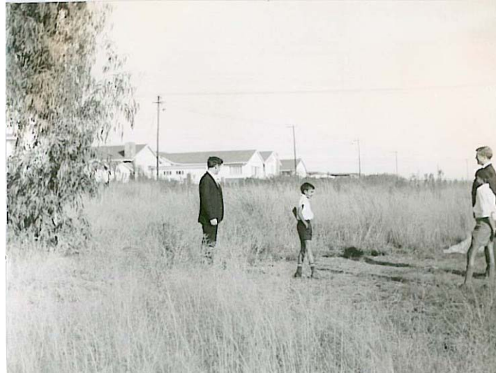
Inspecting the proposed church site In Laudium
