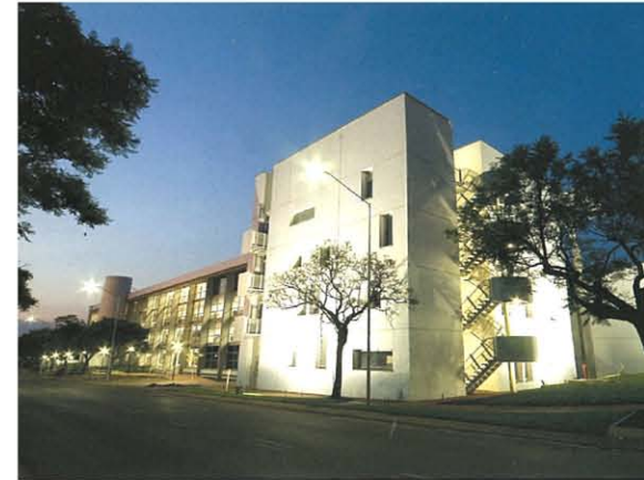
Fig. 6.26: South eastern building mass
