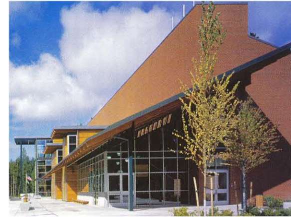
Fig. 6.14: View along northern façade of building
