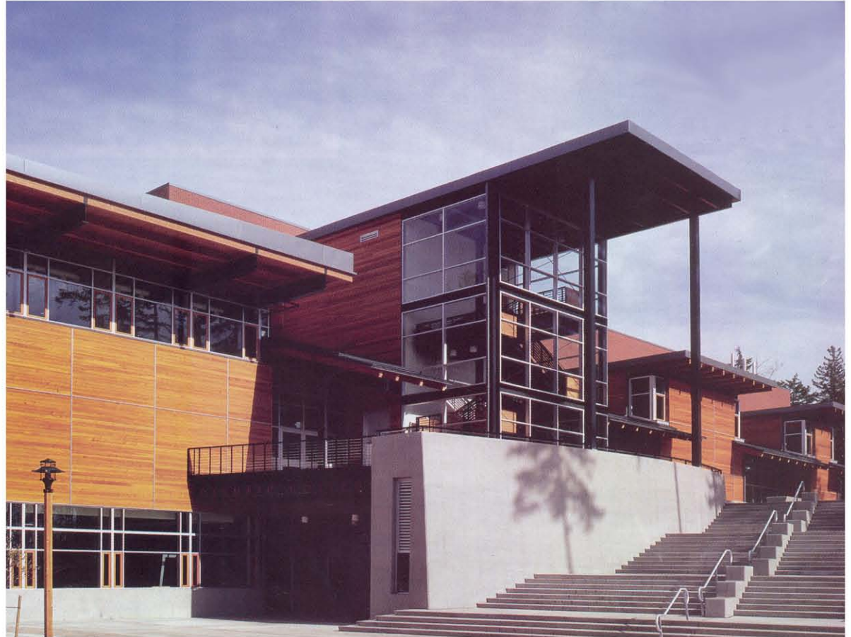
Fig. 6.17: Grand entrance to the school from the drop-off point
