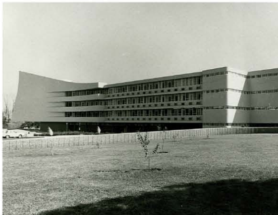
Fig. 7.4: Extensive use of concrete
