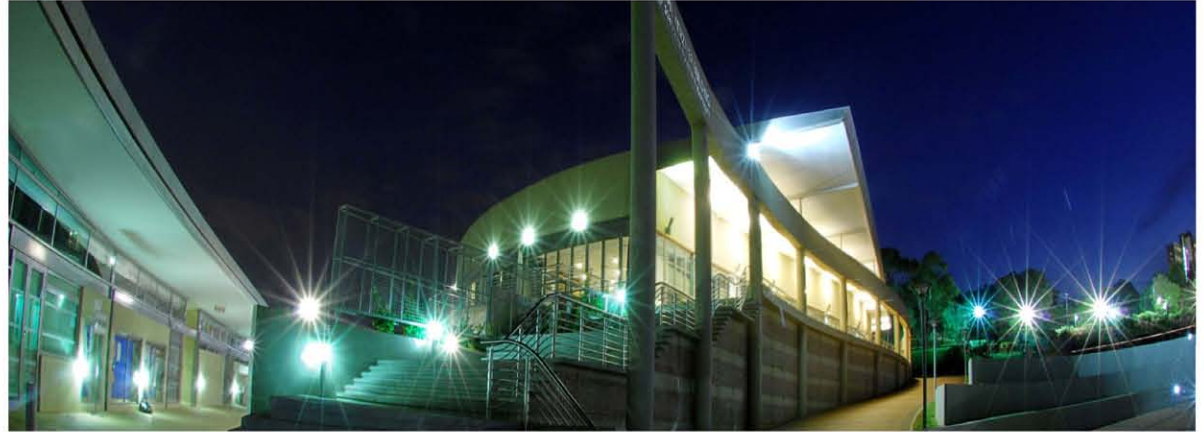
Fig. 6.36: Approach to the main entrance of the Kerzner Building
