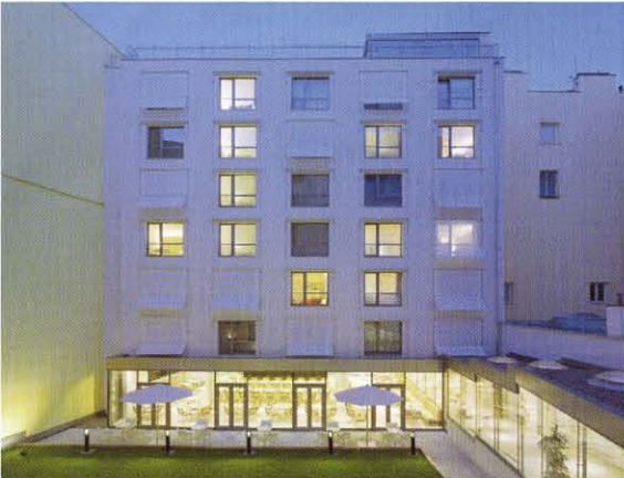
Fig. 6.20: Internal courtyard allowing light penetration
