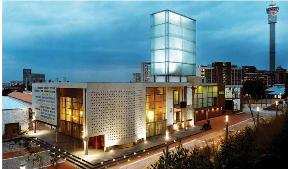
Fig. 6.1: Constitutional Court southern facade
