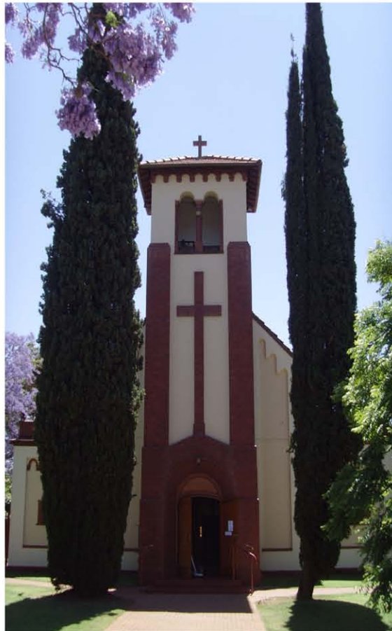
Fig. 5.6: St Wilfred's Anglican Church adjacent to site
