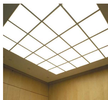
Figure 6.1.11: Stretch ceiling is a suspended ceiling system comprising of two basic components aluminium perimeter track and lightweight membrane which stretches and clips into the track. Additionally, the system can be used for wall coverings, light diffusers, floating panels, exhibitions and creative shapes. Stretch ceilings allow incorporation of all types of light fixtures, recessed lighting, vents and sprinklers by use of an appropriate backend support. The material is unique 0.2mm thick titanium based fully recyclable vinyl. The material can be printed or painted for additional effects, it is waterproof, washable, and resistant to vapor, mold and fire rated class "A". utilized in rehearsal studio .
