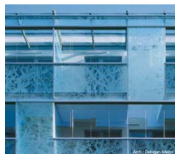
Figure 6.1.10: Screen printed glazing: Double glazed screen printed glass in anodized aluminium window frames Laminated safety glass of 4mm with images screen printed. External windows to be double glazed. Maximum sizes: 1500mm x 3000mm. Utilized in the glazed envelope of the extension to Die Masker staircase seen from the square.
