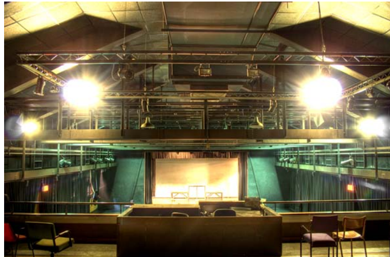
Figure 6.1.1: Interior photograph of Die Masker showing the existing AC duct in roof ridge. By Misra S, May 2008
