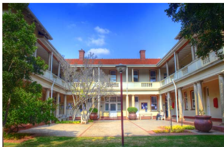
Figure 2.1.9: Panoramic view of the courtyard to the Drama Building (old CBC), by Misra, S, May 2008
