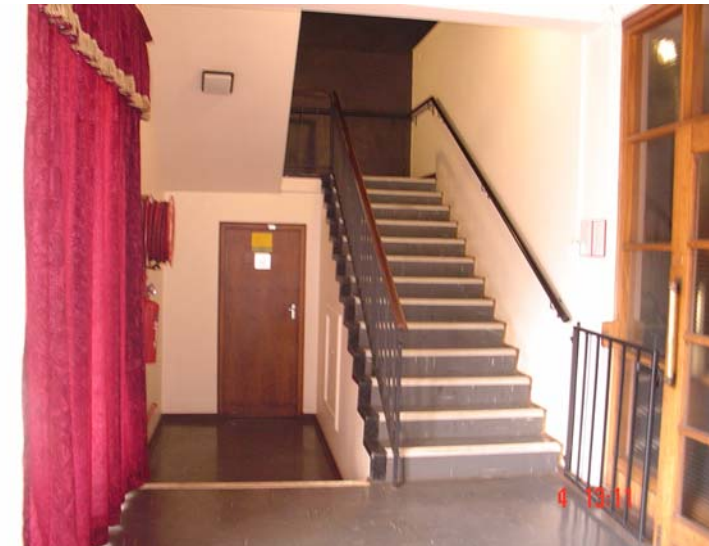
Figure 2.1.19: Interior view of the stairway to the controls level, by Chita M
