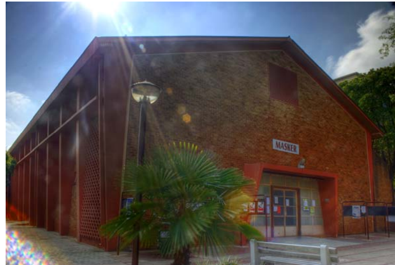
Figure 2.1.16: Die Masker, Existing façade, by Misra. S
