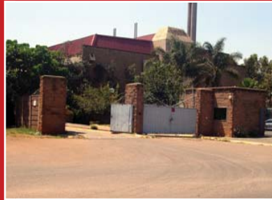
8: Services core buildings (northern elevation)
