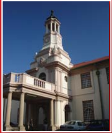
1: Main administration (southern elevation)
