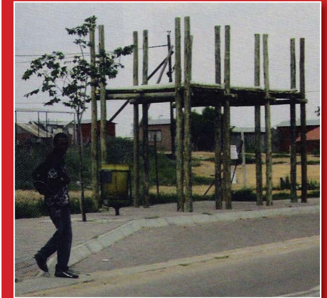
Fig. 5.10: Pick-up and drop-off areas for taxis (Gerald Garner in UGF, Feb. 2007)
