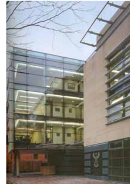
Figure 10: Glass façade representing Transparency in government. Ref: Architect & Builder 2004:22
