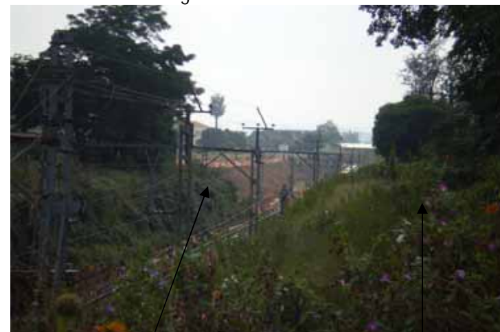
Figure 5: Gautrain Station under Construction
