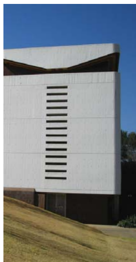
fig. 8.09_existing boukunde building
