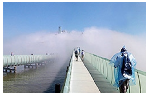
Fig 70. Walkway to entrance of building
