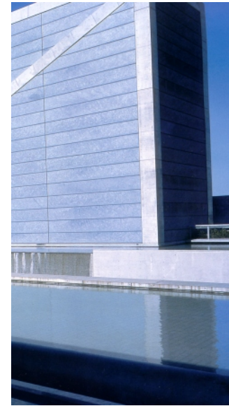
Fig 51. Stone and sheet metal cladding.
