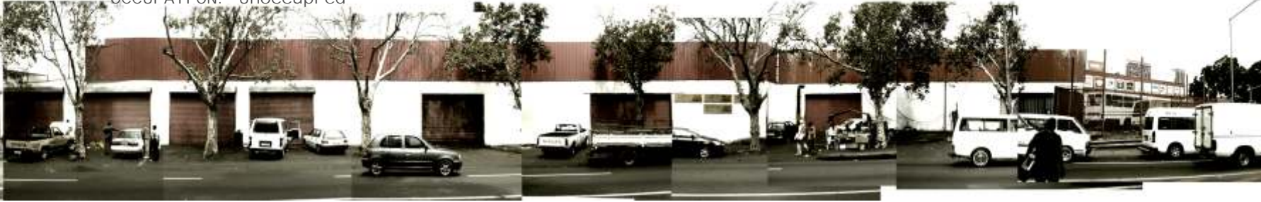
fig 2.43 Building facades on Du Toit Street (western side).
