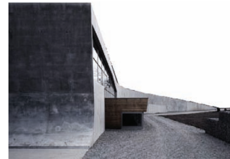
Figure 7.4 Exterior edges of the building
