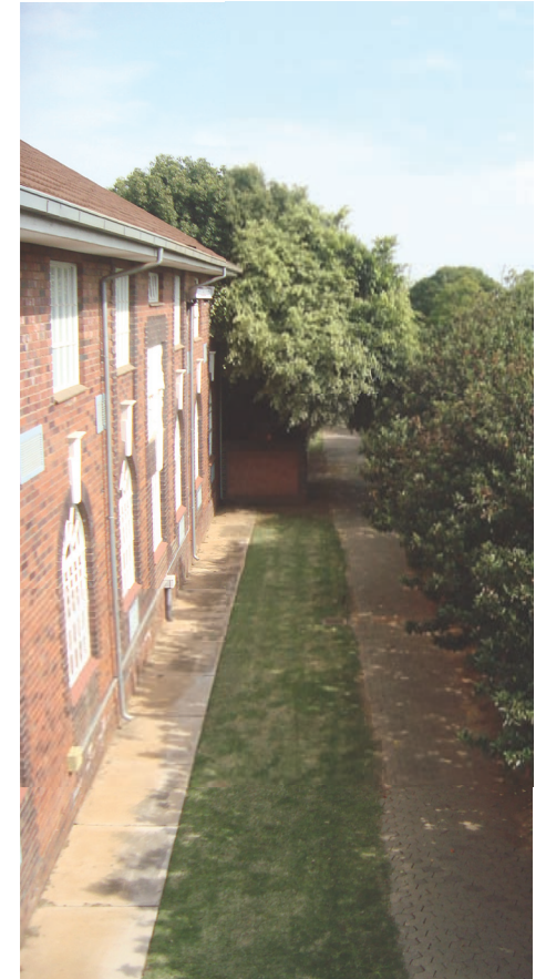
Figure 5.12 Northern facade of Town and Regional Planning Building
