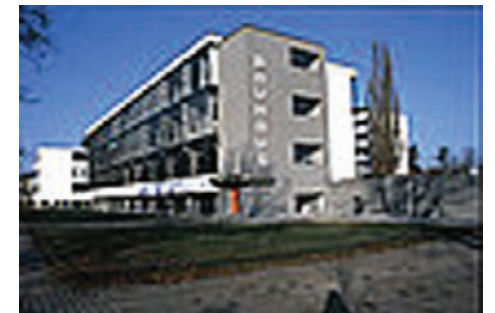
Figure 7.22 Experience on ground level
