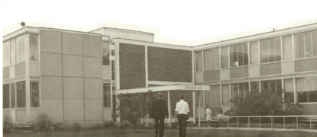
Figure 5.5 Boukunde building view from the north east, 1960.
