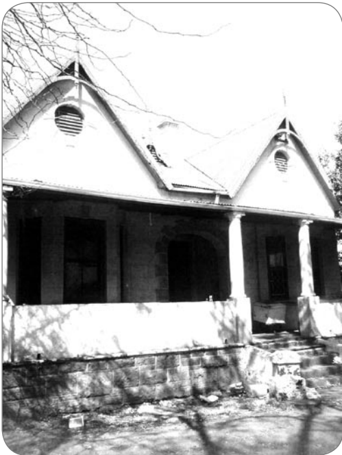
fig. 8.5 front view of building
