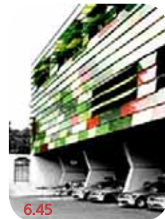
fig. 6.42- 6.45 facade views, berlin fire and police station
