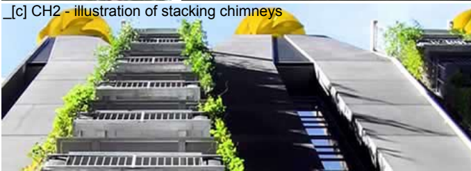
CH2 - west facade timber louvre system powered by photovoltaics fixed on roof
