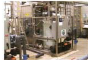
Municipal Drinking Water Township of Tay, OH - 70,000 gpd (263 m 3 /d) Z-BOX M
