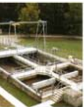
Water Treatment 11.136 m 3 /d ADF* 2-MOD L
