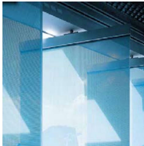
Figure 220: Glass louvres design.
