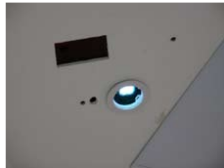
Figure 236: Brooklyn Mall ceiling.
