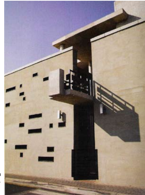
Figure 148: Baragwanath Transport Facility.
