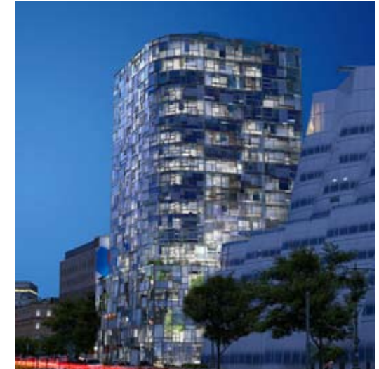
Figure 86: Glass curtain wall on south façade.
