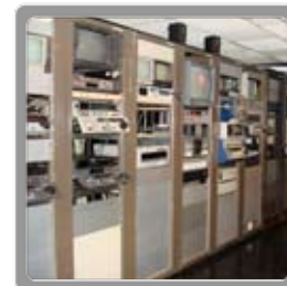
Figure 101: Server room and equipment store, The Video Lab, LA Film School.
