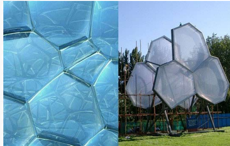
Figure 174: Water Cube façade prototype.
