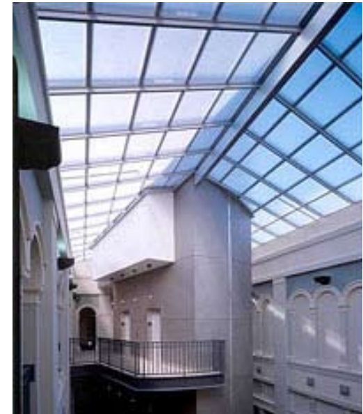
Figure 191: Nanogel® used in glass roof.
