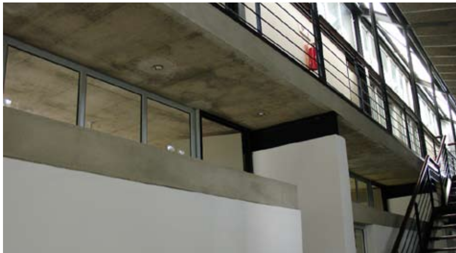
Figure 188: Internal light shelf.
