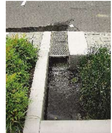
Figure 199: Networked sidewalk storm water system, Portland Bureau of Environmental Services.
