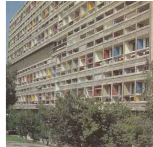
Illus. 5 Unite d'Habitation, Marseilles, Le Corbusier, 1952-55, showing his use of exterior colour in his insertion of primary hues into recesses and around apertures in the facade. (PORTER 1982: p.20)
