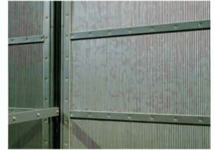
66 MINIWAVE CORRUGATED STAINLESS STEEL SHEETING, PROFIL ARBED HEAD OFFICE, LUXEMBOURG, BOHM AND MINKUS ARCHITECTS INTERNATIONAL IRON AND STEEL INSTITUTE : 1997
