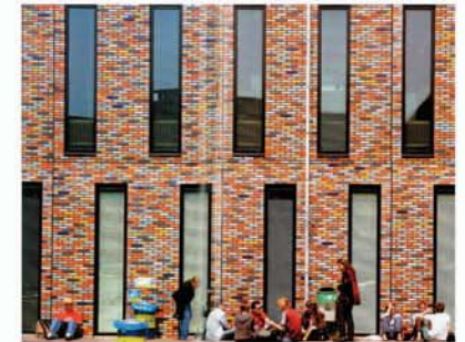
67 BRIGHTLY COLOURED GLAZED BRICKS, RAINBOW ALLIANCE, HOLLAND, DE TWEE SNOEKEN ARCHITECTS, 2004 BRICK BULLETIN : 12/2006
