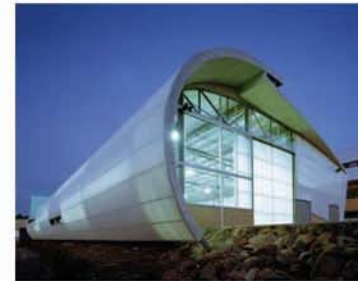
52 CURVED TRANSLUCENT SHEETING POLYMER ENGINEERING CENTRE, VICTORIA, AUSTRALIA BELL, V. B., ET AL. : 2006
