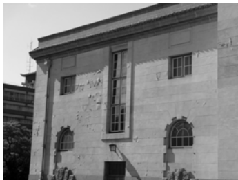
Fig. 45 Plaster and paint finish of western facade (Author 2006).
