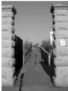
Fig. 27 Pretoria Station Bridge to Salvokop from the station. (Author, 2006)
