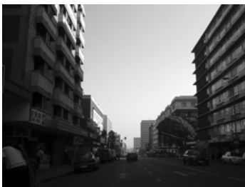
Fig. 14 A typical street edge condition of Paul Kruger Street south (Author, 2006)
