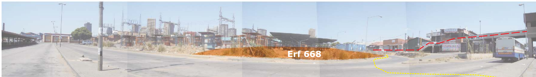
Figure 4.9: View of erf 668 and electrical substation from Belle Ombre bus station
