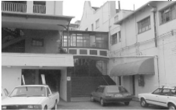
Figure 6.12: South-Eastern view of bridge
