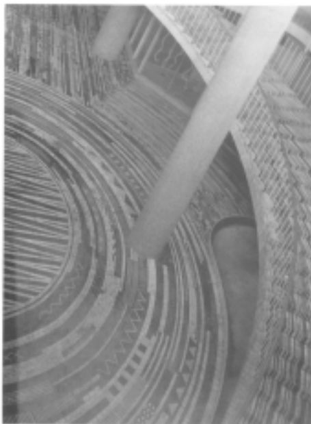
Figure 10.2: Polley's Arcade, Pretoria - Norman Eaton. Stairwell detail. 1953.
