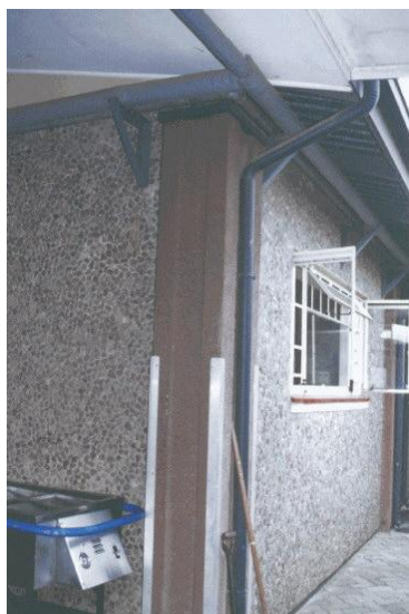
Figure 25 – A view of the precast structure of the dormitories (photograph courtesy of Little Eden Society)
