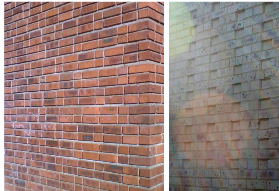
Figure 77 – Photographs of various brick bonds (photos by author)
