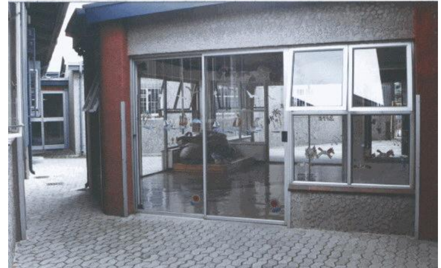
Figure 26 – A view of the sun room in yellow wing (photograph courtesy of Little Eden Society)
