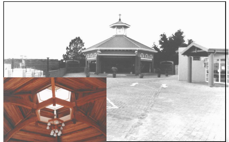
Figure 28 – An external view of the chapel as well as a close-up of its timber ceiling (photographs by author)
