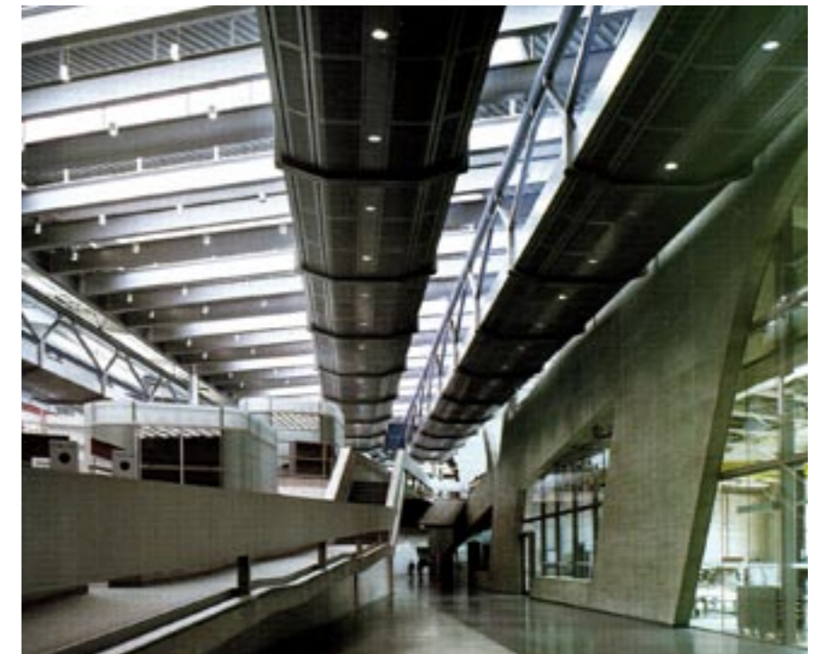
Fig.63: Inside walkway showing conveyor belts suspended from the ceiling.
