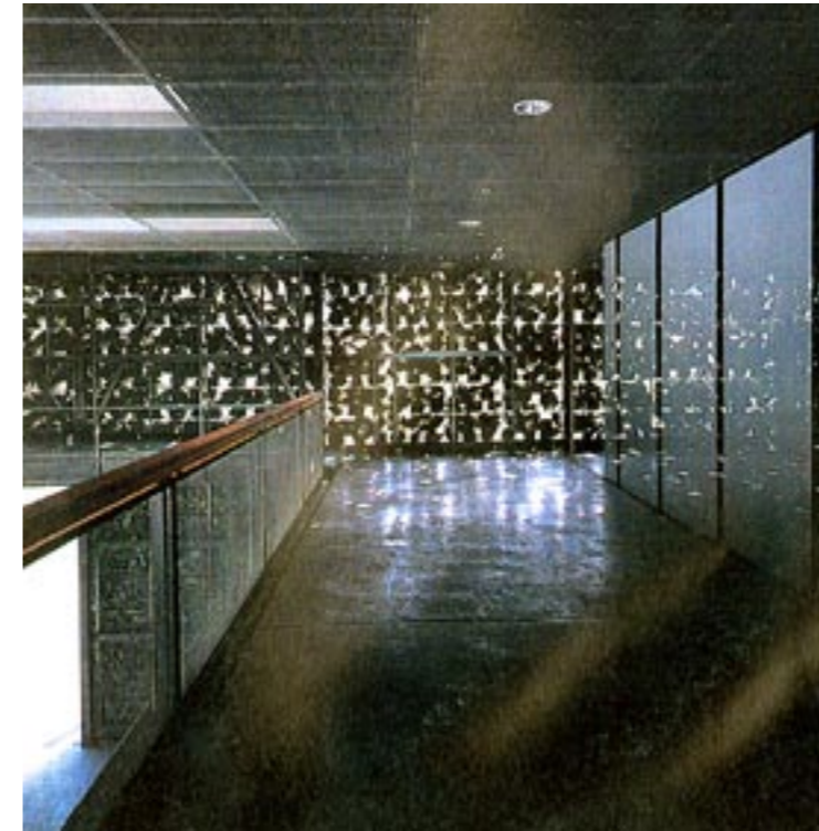
Fig.59: Interior view of the Dominus Winery showing sunlight penetrating the gabion wall.
