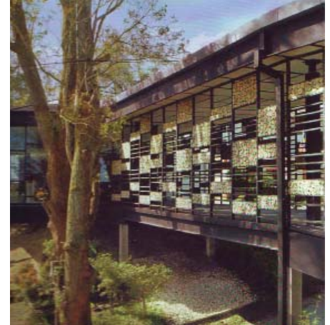
21. BOH Visitors Centre - View along East Facade
