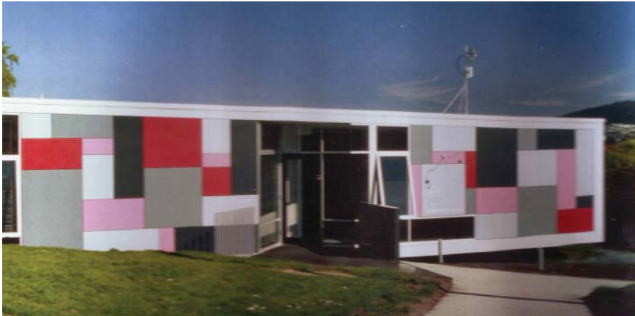
24. Clarence Family Day Care Offices - North Facade
