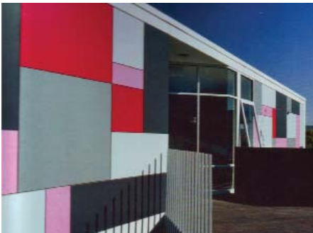
25. Clarence Family Day Care Offices - Detail of Fibre Cement Sheeting
