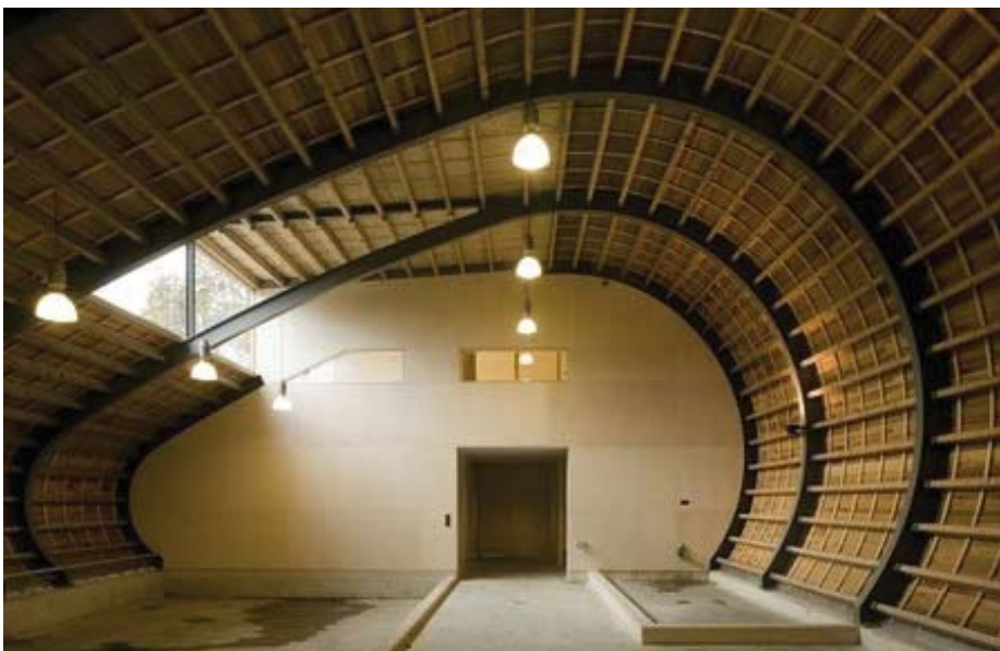
122. Sheep Stable - Internal View & Clerestory Window Detail
