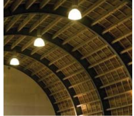
120. Sheep Stable - Lighting Detail
