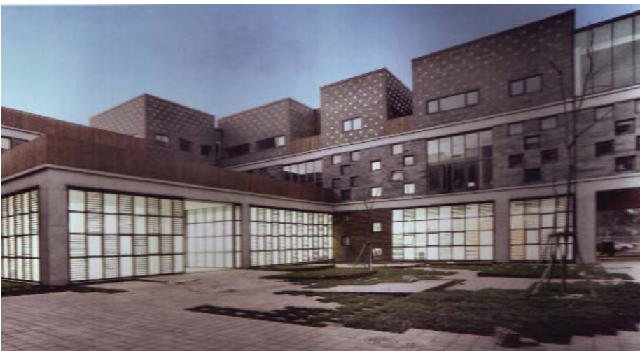
23. UF Soft R&D Centre - Main Entrance & Second Courtyard
