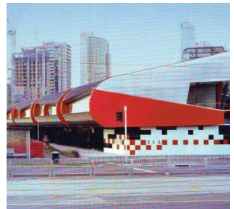
117. State Emergency Services Headquarters - View from Street
