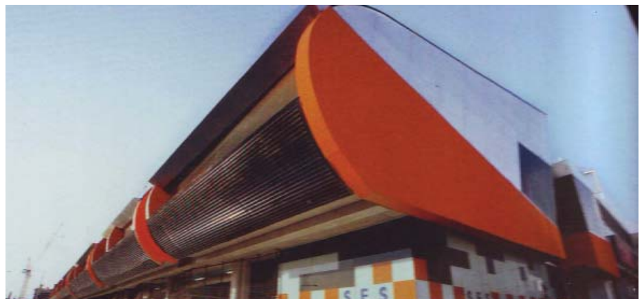
118. Emergency Services Headquarters - Fracturing and Colour Use
