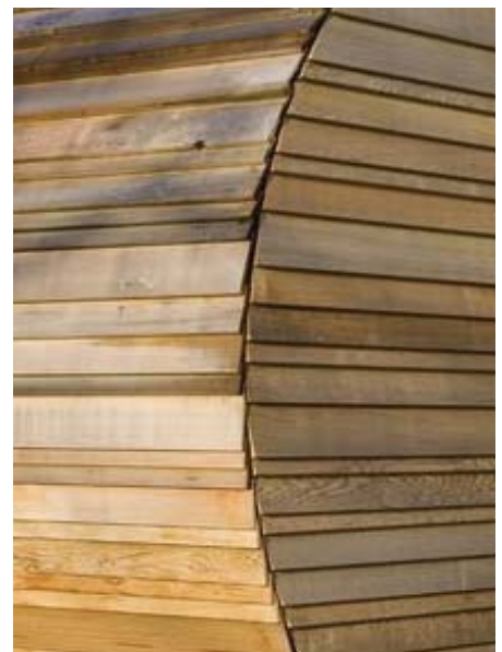
123. Sheep Stable - External Cladding Detail
