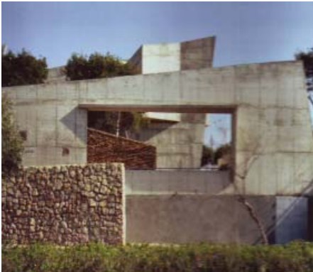
11. Palmach Museum of History - detail of concrete and limestone walls
