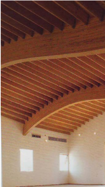
114. Commercial Building 3555 - Interior Ceiling
