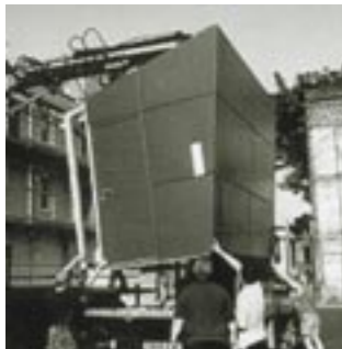
Figure 156: Installation of Bradbury St. vendor stalls.
