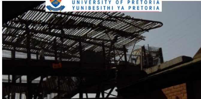
Fig 7.11: Bridge roof to herb market
